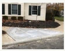
Parking lot curbs were fixed and the old handicap ramp removed on November 30. This work needs to precede resurfacing the parking lot in the spring.
