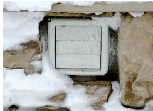
Clothes dryer vent should not be covered with snow
