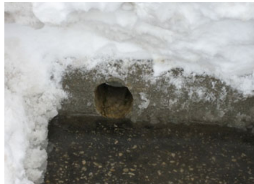
Curb drain from sump pump and down spouts
