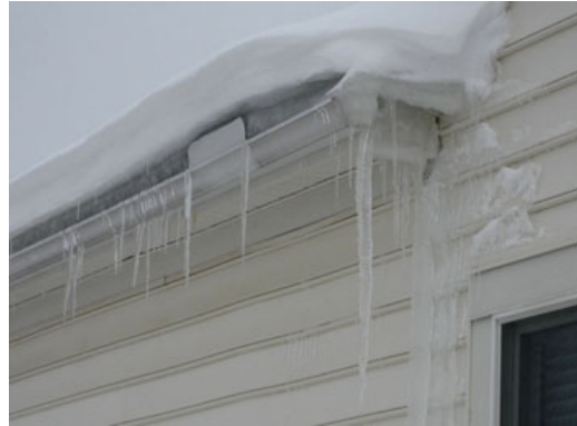
Ice dam blocking water run off
